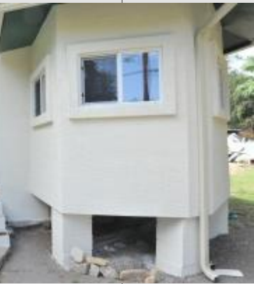
Arizona Silver Belt Perez show off their new home major rehabilitation thanks to Community Housing Services.
